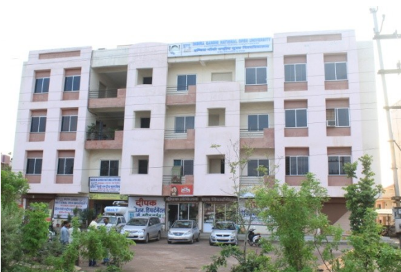
NEW BUILDING OF RC RAIPUR-35
